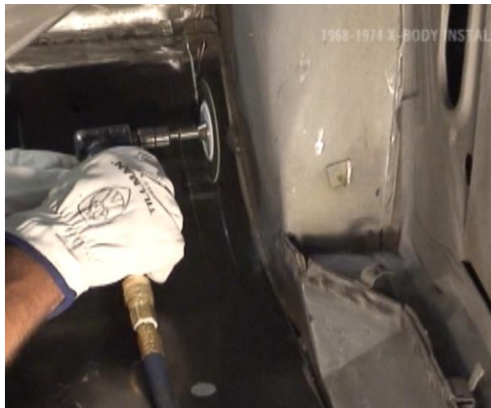
Figure 14 – Cut 1-1/4" Marked Lines
