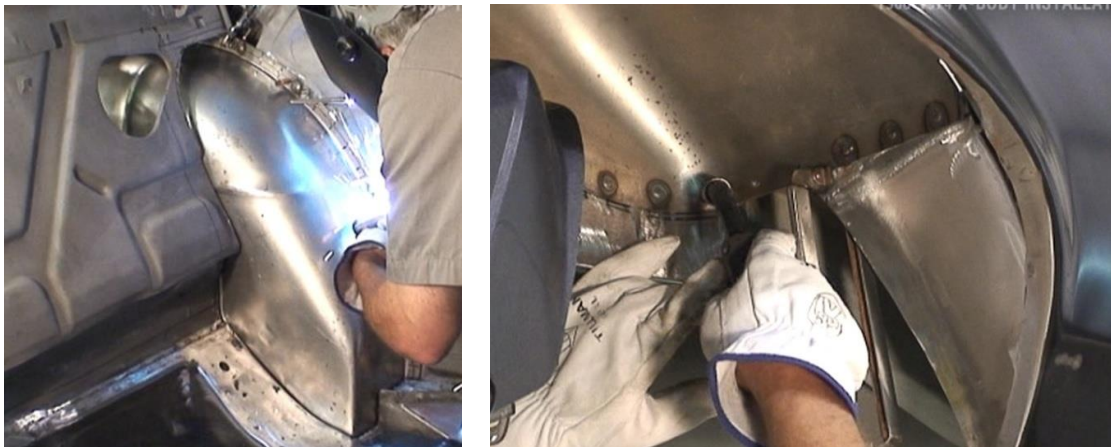
Figure 29 – Welding the Mini-Tub
