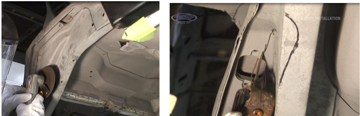
Figure 17 – Cutting along the Framerail
