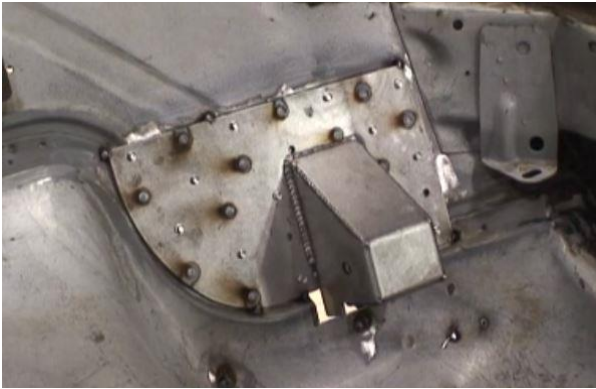
Figure 5 - Plug and Tack Weld in Place
