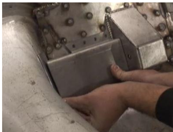
Figure 10 - Fit the Inner Brace and Tunnel Doubler
