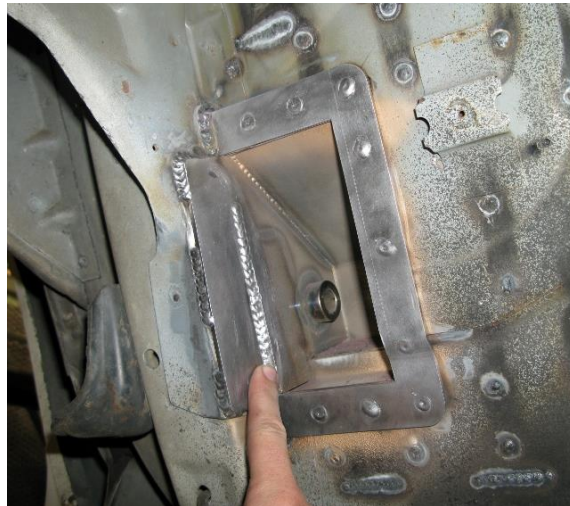
Figure 17 - Finish Weld Flange & Close-Out
