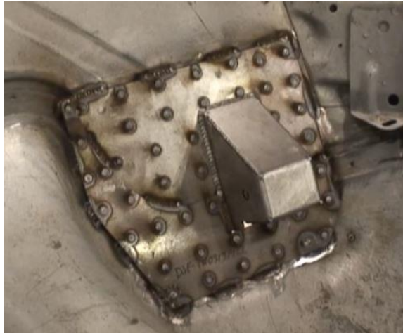
Figure 9 - Finish Weld Lower Doubler Plate
