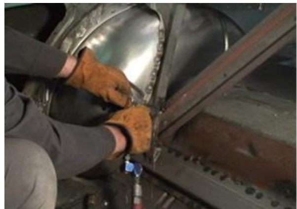
Figure 15b - Welding Modified Brace
