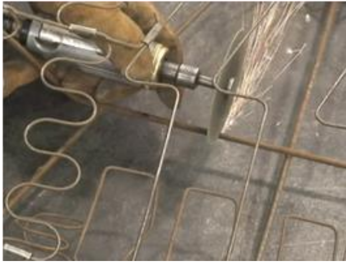
Figure 26 – Cutting the Cross Bar at the 2-1/2" Mark
