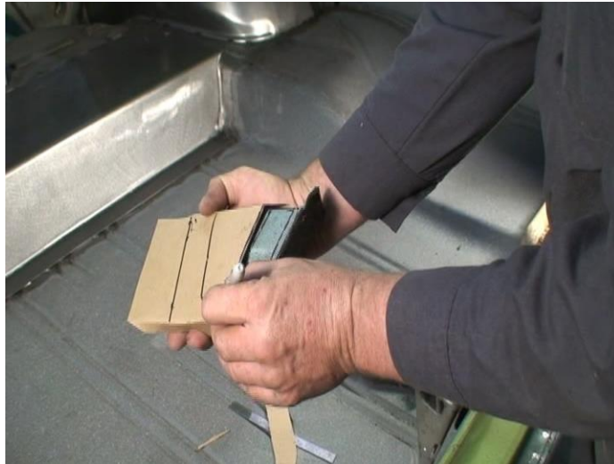
Figure 16 - Comparing Cardboard Template to Factory Trunk Flange
