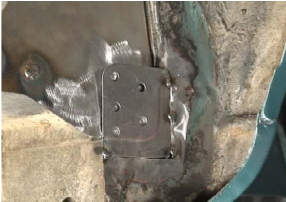
Figure 14a. Welding Fabricated Front Lap Flange
