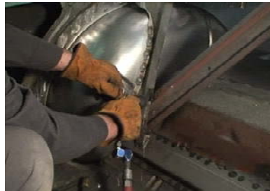
Figure 15b. Welding Modified Brace
