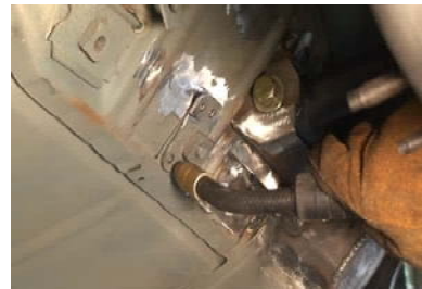
Figure 21c. Welding Anchor (Supported by Anchor Bolt)
